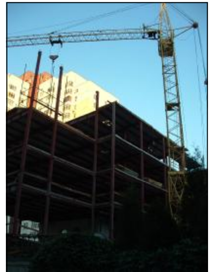
Crane working on 5-storey addition at KTS
